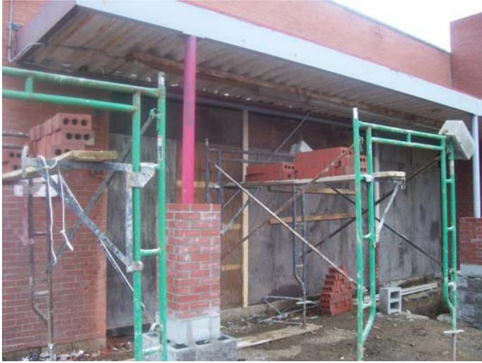
The rehabilitation plan included updating the façade. Existing steel supports were wrapped with brick and block
