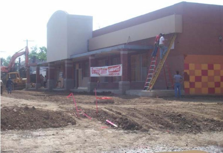
Framing complete, the tower now has stucco in place, and work begins on ancillary signage boards. The building exterior begins to finally take shape.
