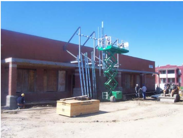
As we freshen up the façade, we also looked at building signage. Here, the steel framing for a new tower is being put in place by Empowerment Zone business Baker Welding.
