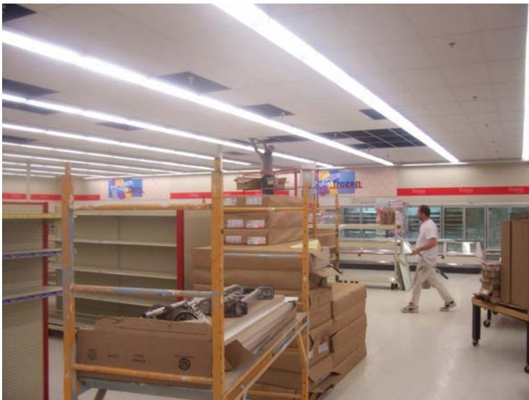
As flooring is finished, Save-A-Lot begins bringing in shelving units. Note the ceiling tile has been dropped, and interior store signage and branding is going up.
